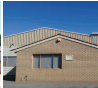
U2-15 Vale Street Malaga 370m 2 approx Office/Warehouse fully fitted out (previous use Laboratory)
